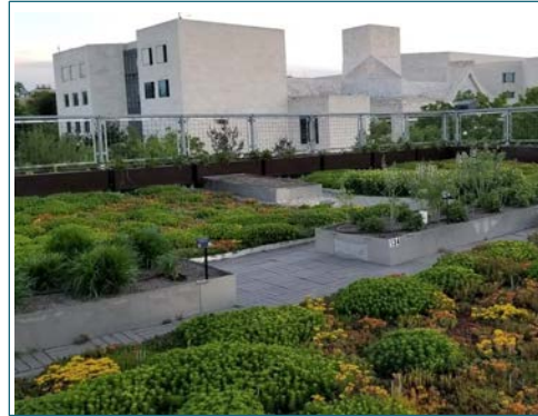
Figure 3: LEED encourages sustainable strategies to combat the heat island effect like green roofs.
